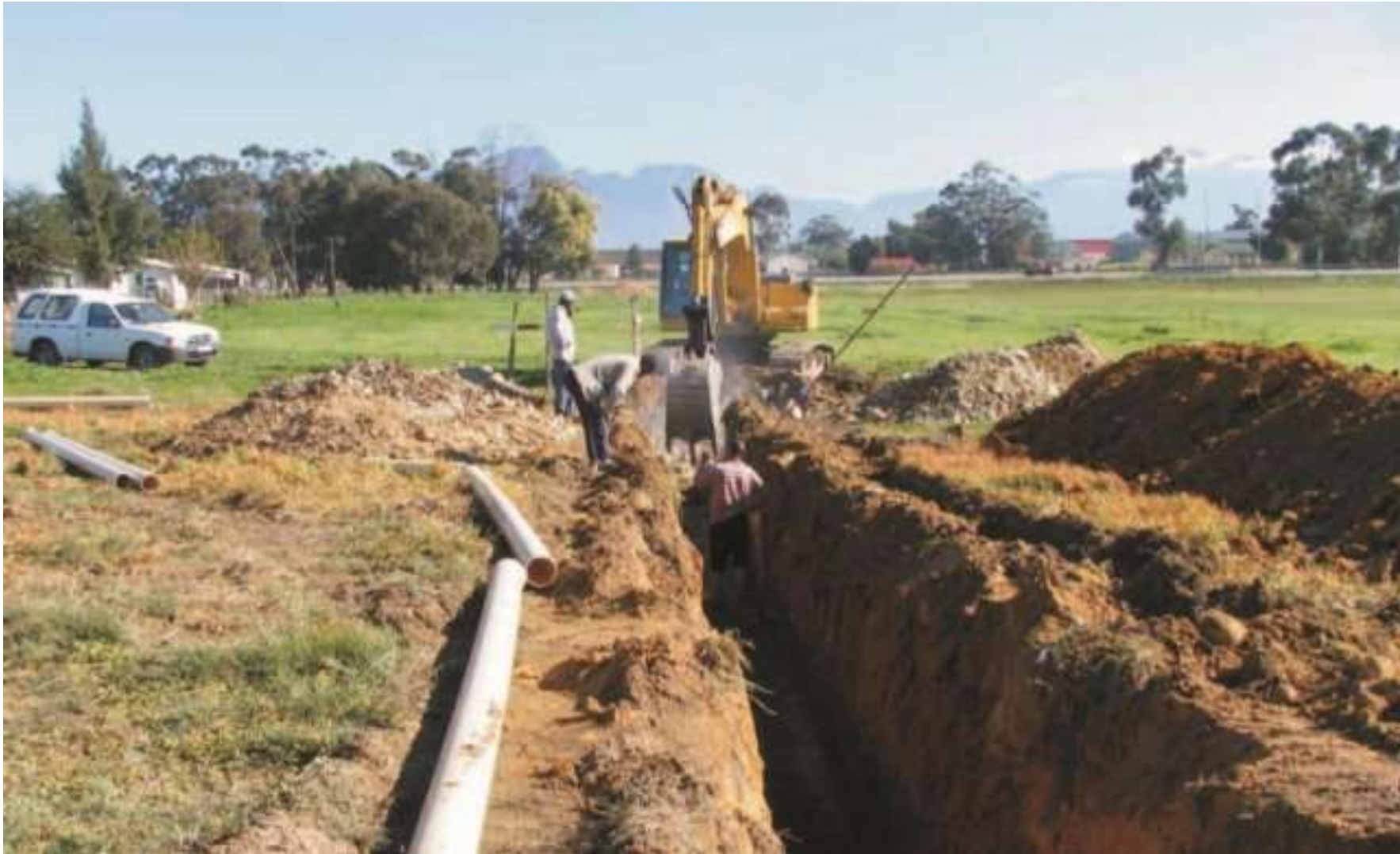
Replacement APC to PVC Pipes in Ward 4
