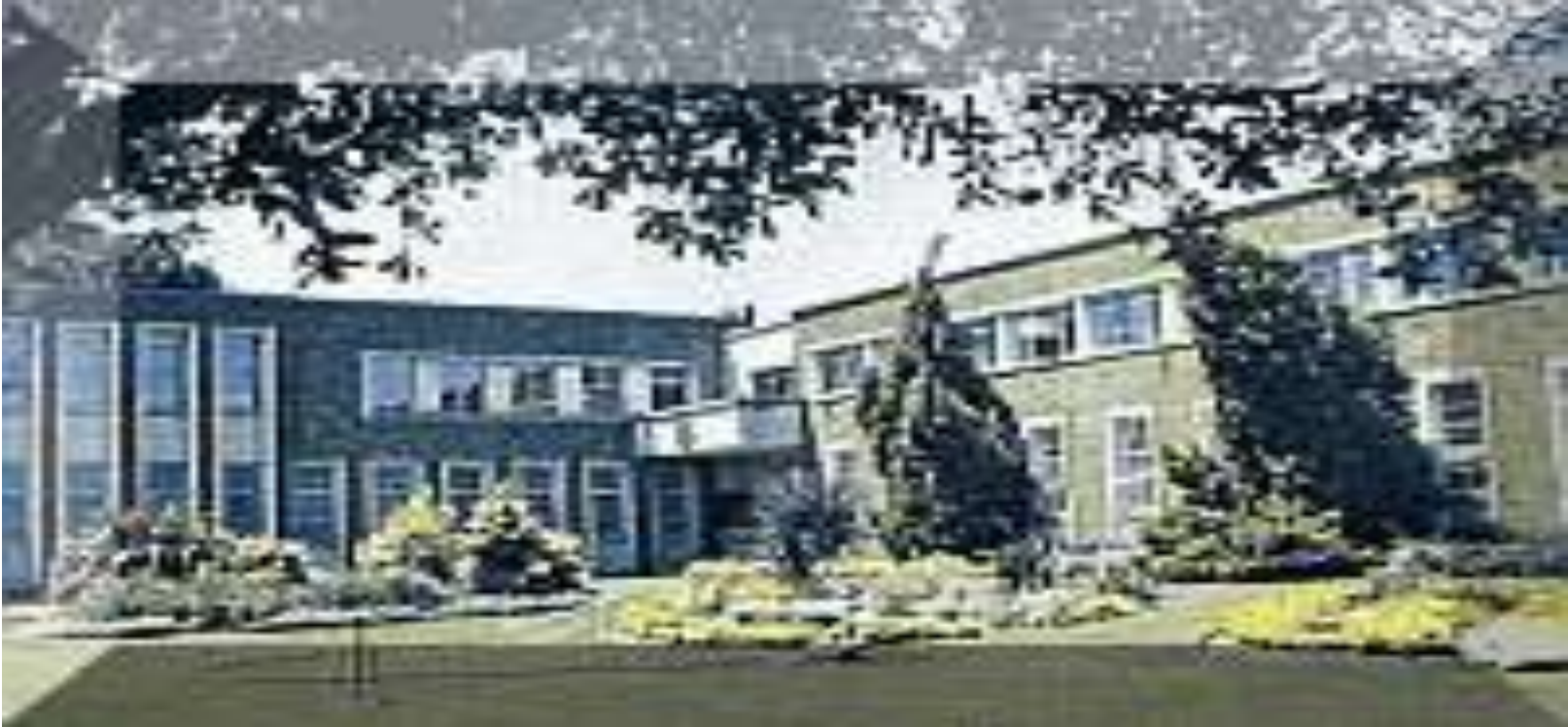
Main Municipal Building
